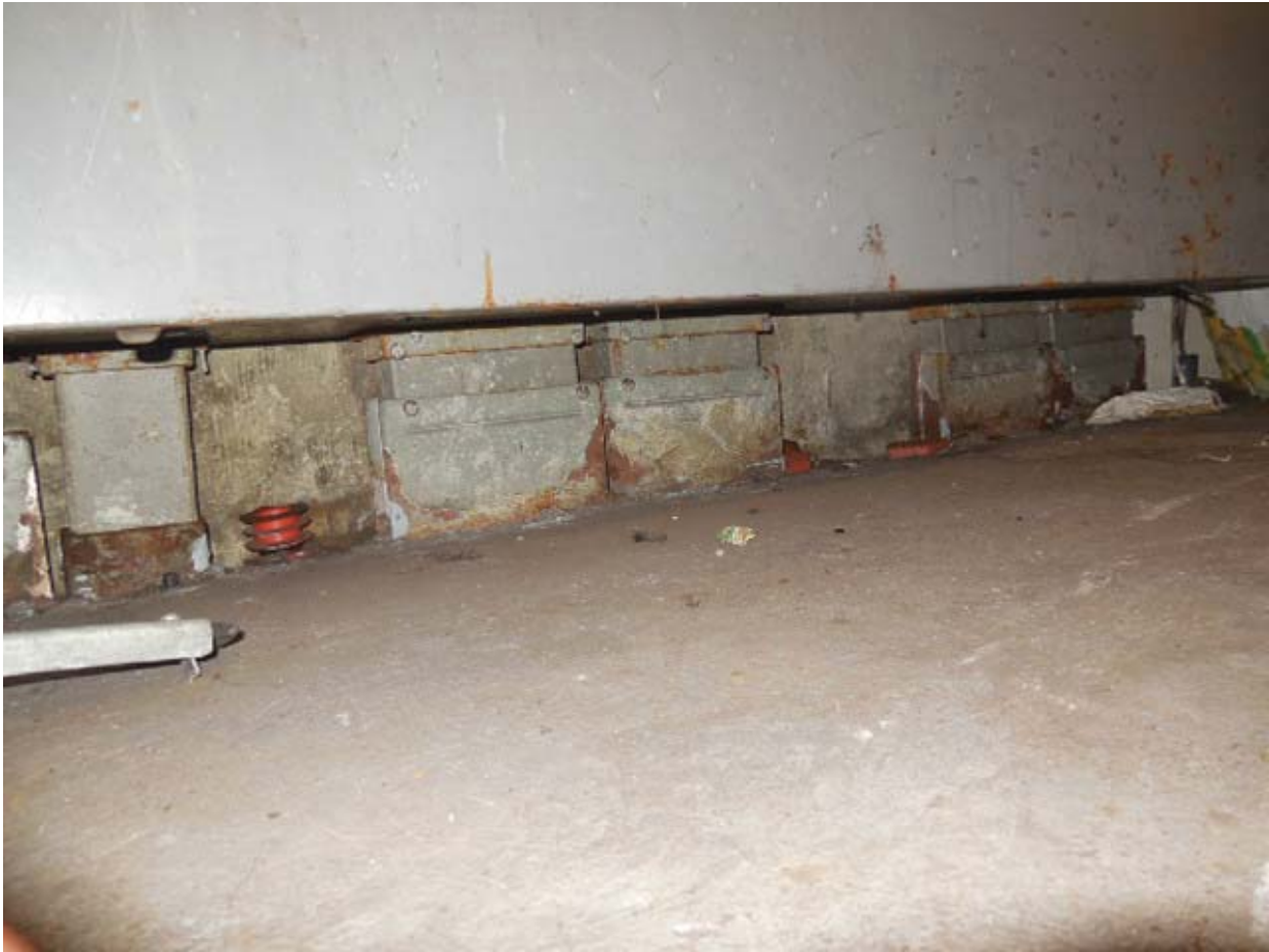
Picture 11: F04 Waterfront – Panel MESS-1 shared trough in Room C206
