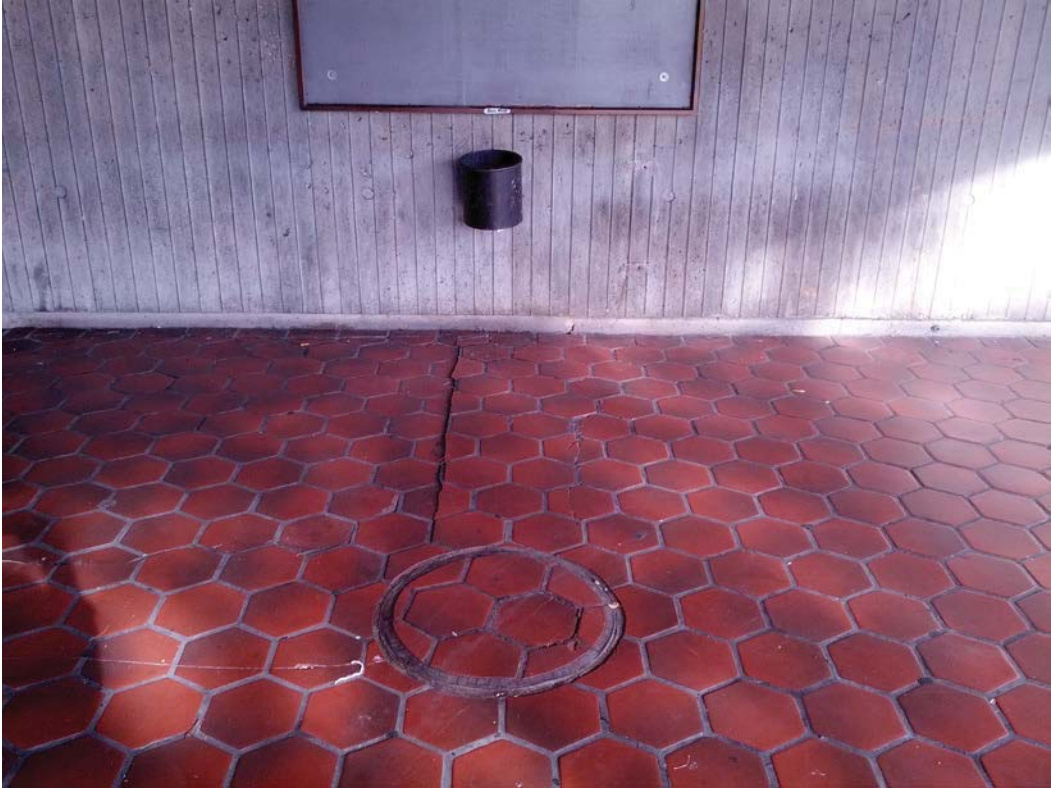
Pictures 1&2: F06 Anacostia (South) – Manhole near eastern entrance gate
