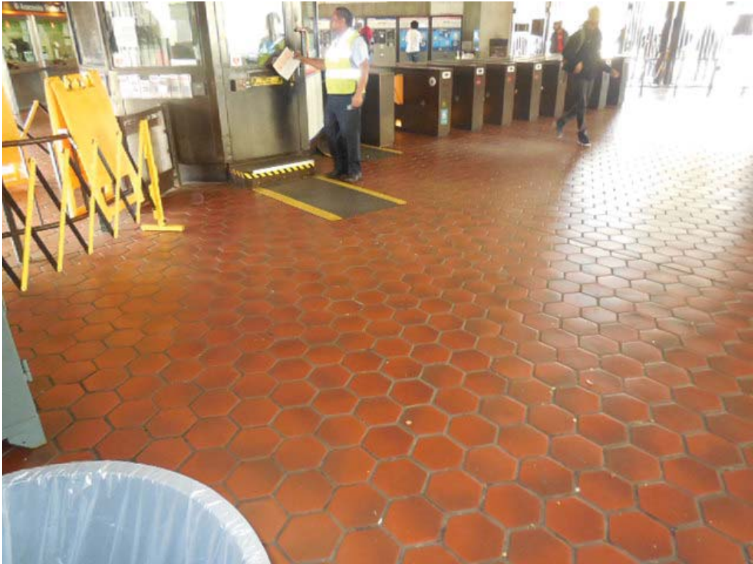
Picture 3: F06 Anacostia (South) – No handholes in mezzanine
