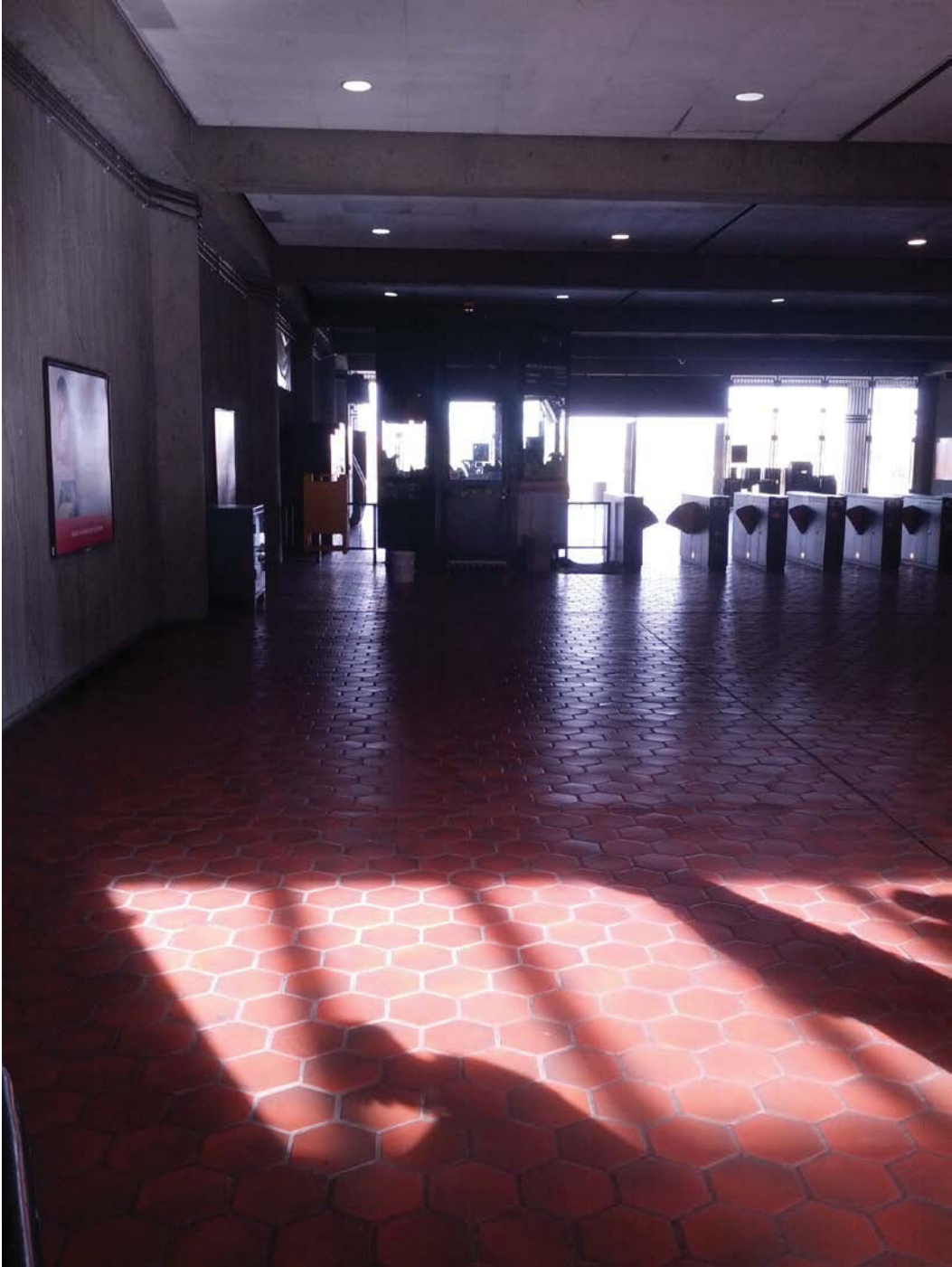
Picture 1: F06 Anacostia (North) – No handholes in mezzanine
