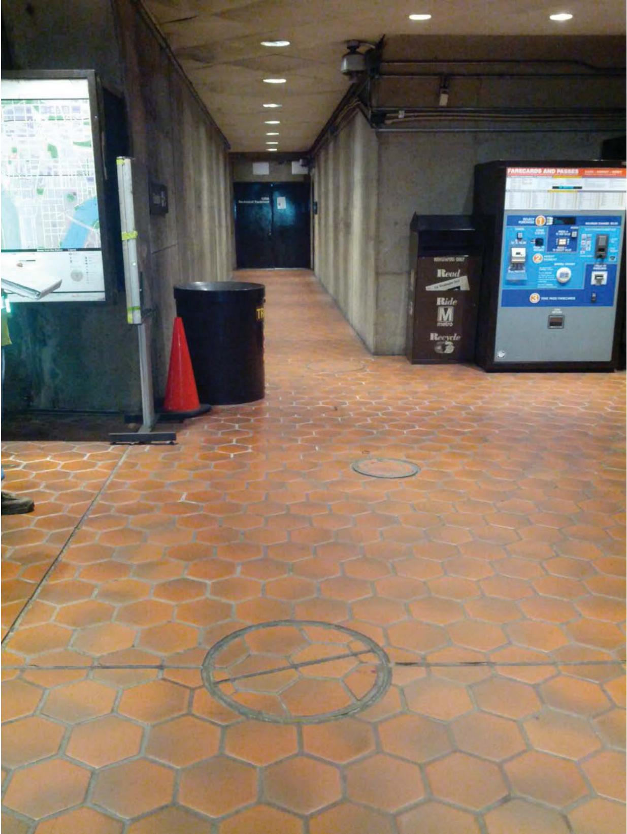
Picture 1: F04 Waterfront – Mezzanine manholes
