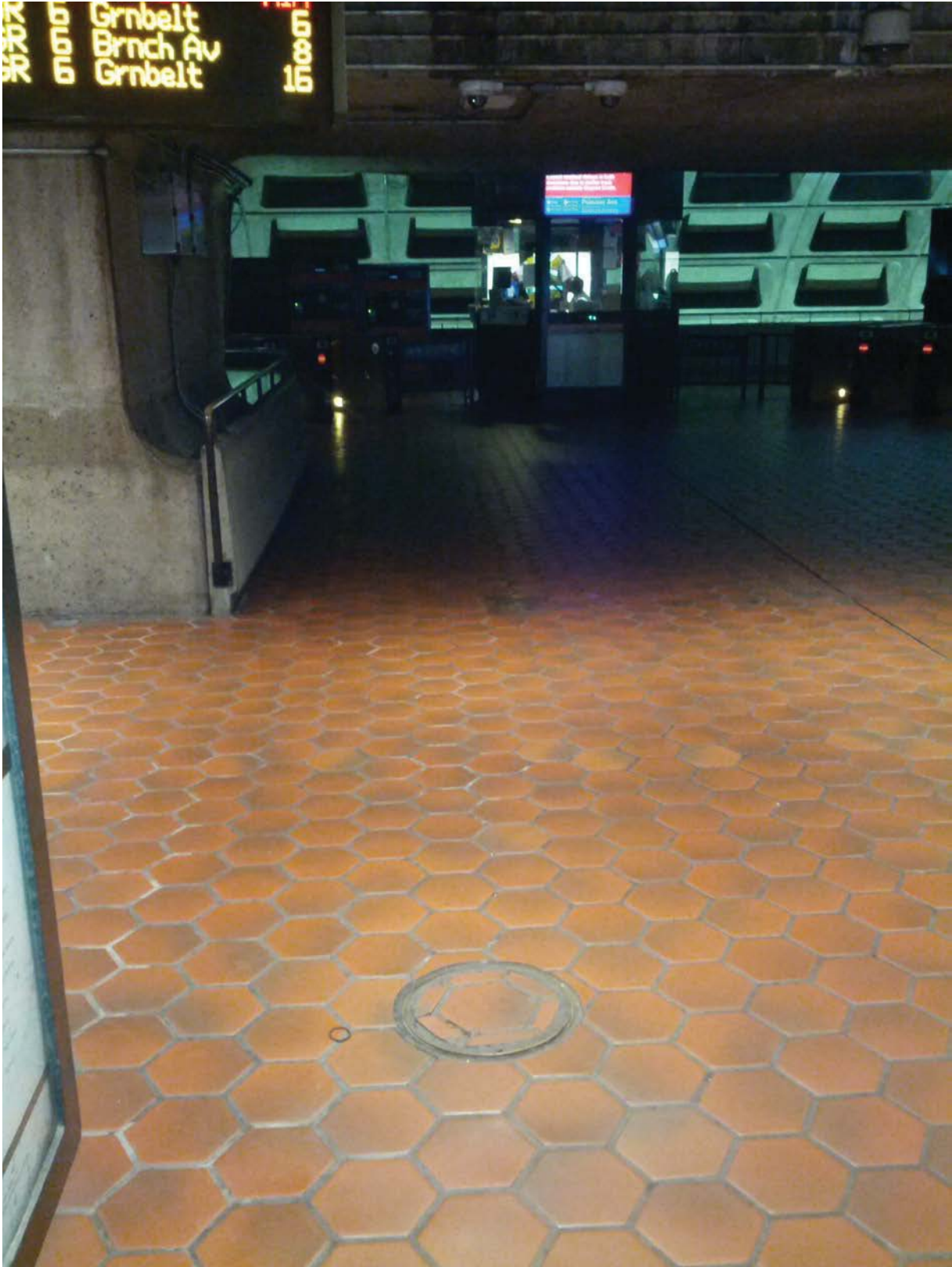
Picture 3: F04 Waterfront – Mezzanine manhole-2
