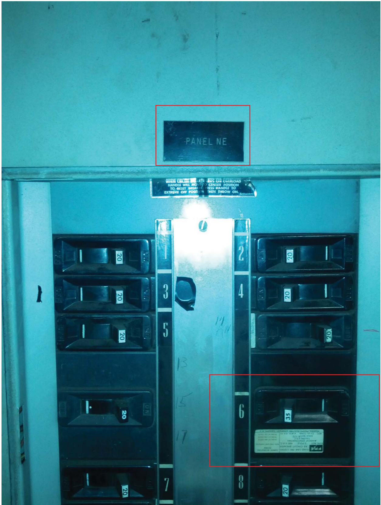
L'Enfant Plaza North Photo #14 – Panel NE - Circuit #6 is breaker for Panel NEZ
